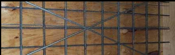
Before pouring concrete, note rebar
